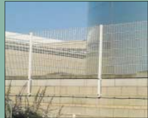
Compound wall and fence topping protected by WallSecure™ detection system
