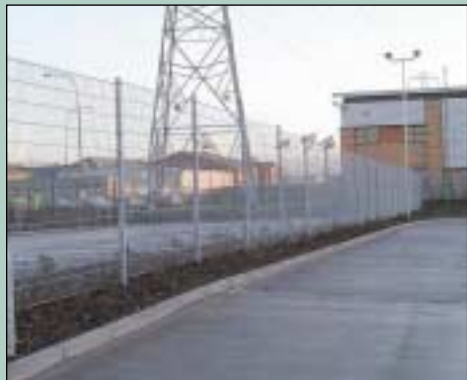
Logistics compound perimeter fence protected by FenceSecure™ detection systems
