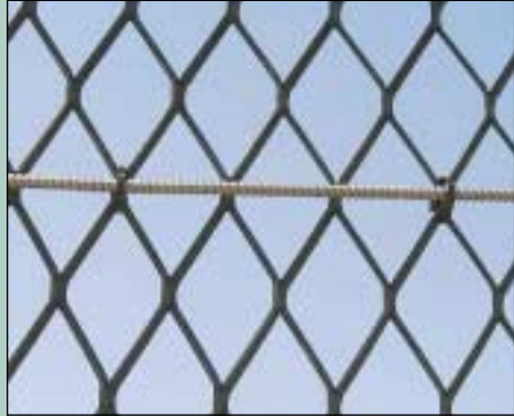
Expamet fence protected by FenceSecure™ detection system
